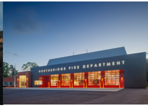
Station 1 Northbridge, MA
