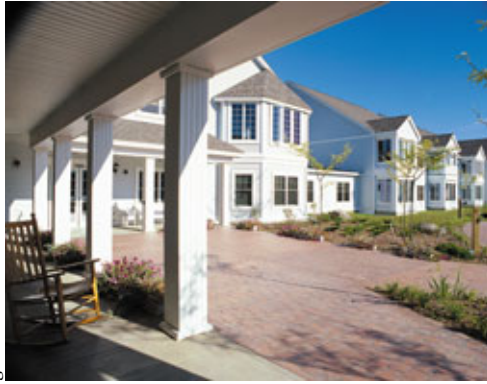
gablers at east mountain
